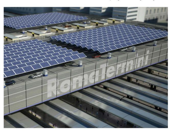
necessary to reach the support avoiding a downwards deflection that would prevent the reaching of the correct height. All the steel structure has been assembled and launched from the top of the station, without interfering with the below train traffic.
